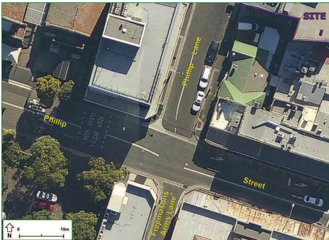
Figure 4: Phillip Street /Phillip Lane/ Freemasons Arms Lane Intersection
