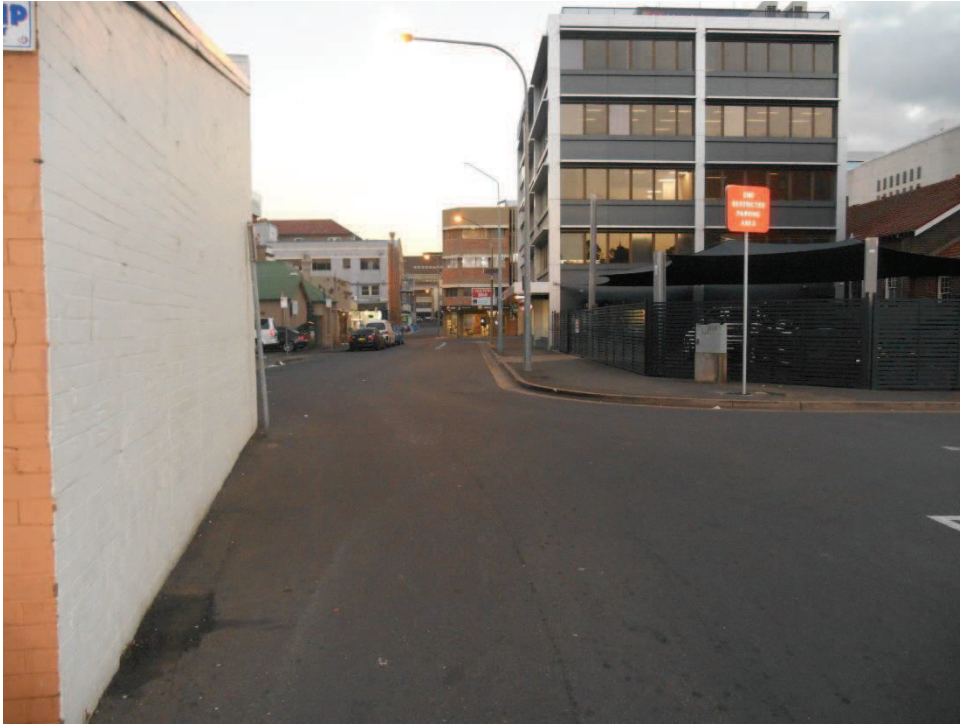
View looking south along Phillip Lane towards Phillip Street providing a more detailed view of the lane geometry.
